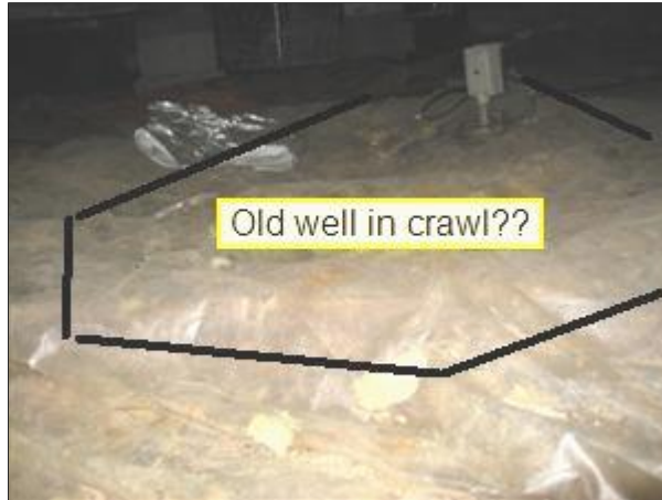
2.6 Picture 2 in crawlspace under new addition
