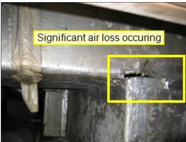
6.3 Picture 4 crawlspace new addition
