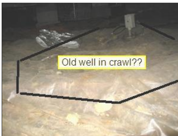
2.6 Picture 2 in crawlspace under new addition
