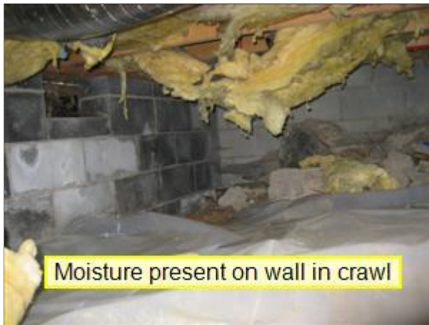
1.0 Picture 5 crawlspace under kitchen
