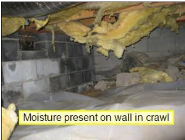
1.0 Picture 5 crawlspace under kitchen
