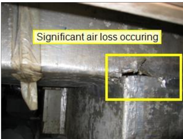
6.3 Picture 4 crawlspace new addition
