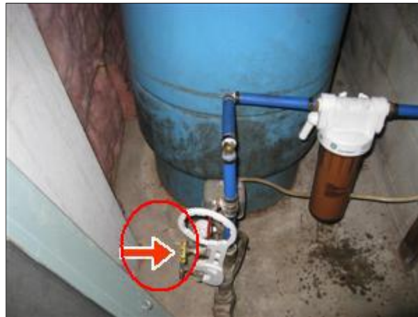
4.3 Picture 1 In basement
